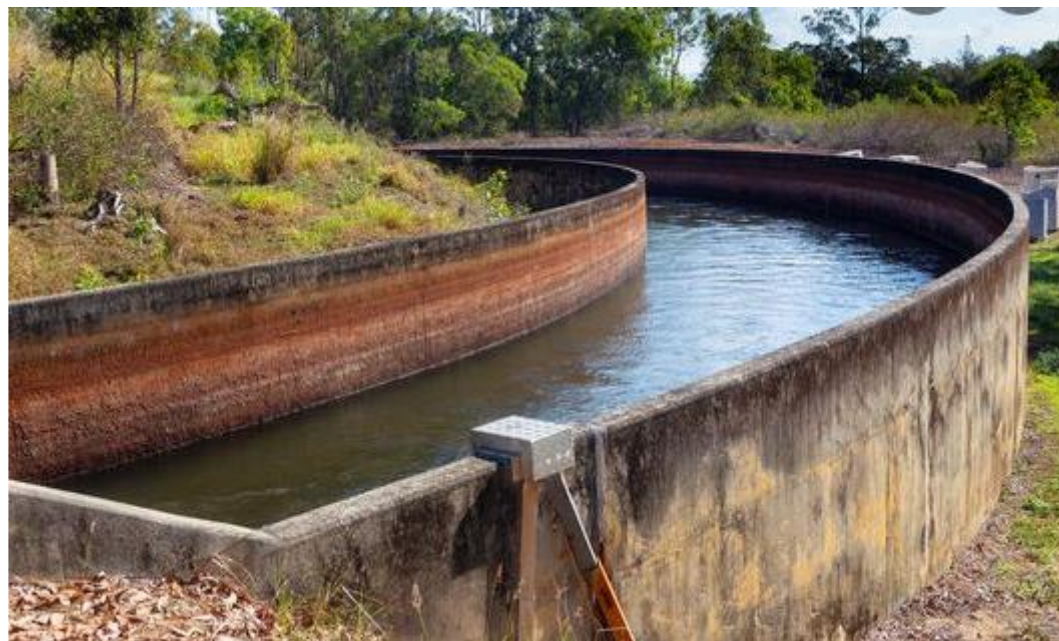
Tinaroo Falls Dam; Bench Flume Constructed by IWSC (1950s)
