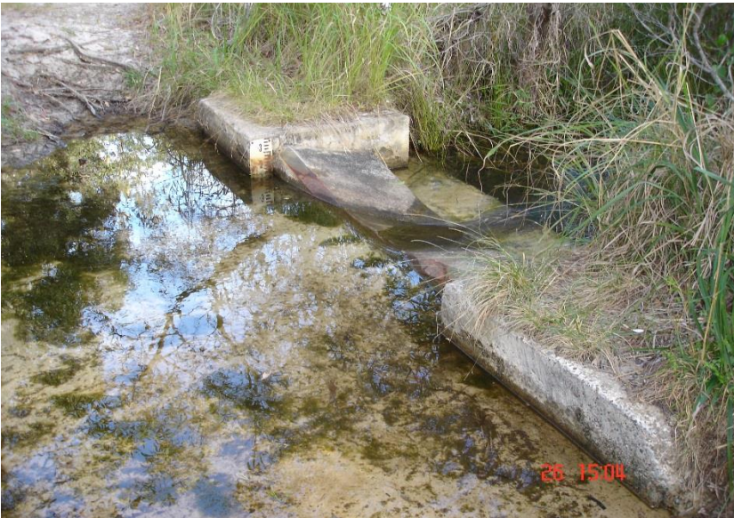
Surface Water Measuring Flume
